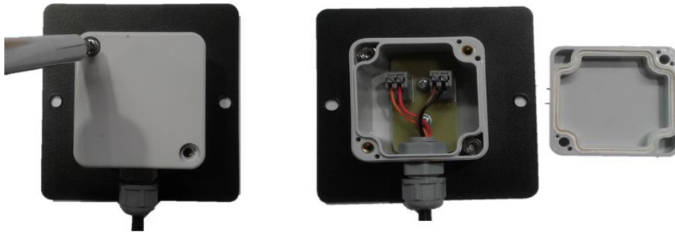
Fig. 9 – Opening the back of the wallswitch
