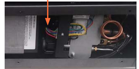
Adjustment screw burner pressure
